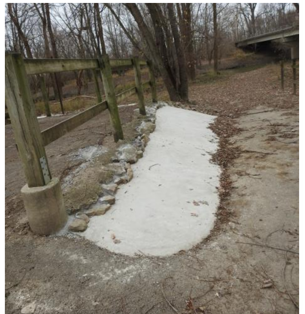
Parking lot repairs at Rainbow Bend were needed to fix erosion issues caused by Wabash River flooding
